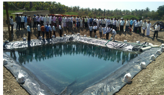
Construction of Farm pond and lining with the Geo membrane polythene
