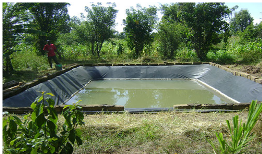
Construction of Farm pond and lining with the Geo membrane polythene
